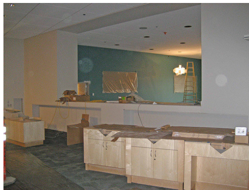
Photo of the Mastodon case under construction.
